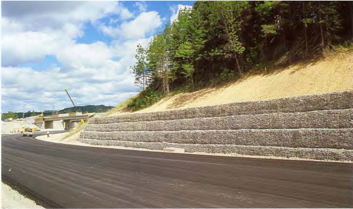
Figure 15.9: Maccaferri Canada Ltd., Terramesh System (Gabion) – Wall/Slope, Medium Performance, Low Appearance Wall.
