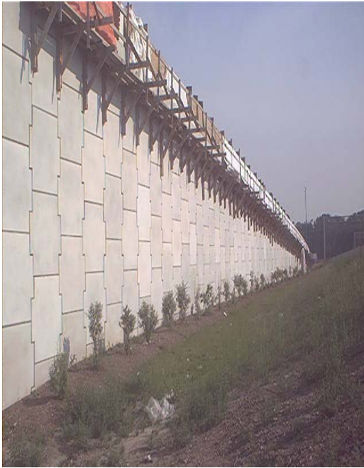
Figure 15.3: Reinforced Earth Company Ltd (RECO), Cruciform – Wall/Slope, High Performance, High Appearance Wall.
