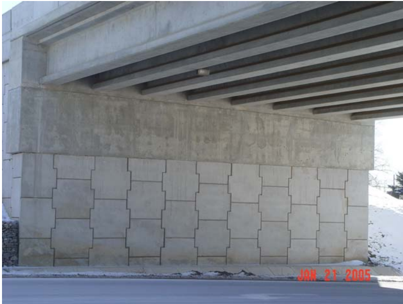
Figure 15.2: RSS False Abutment (Integral) with RSS Wingwalls.
