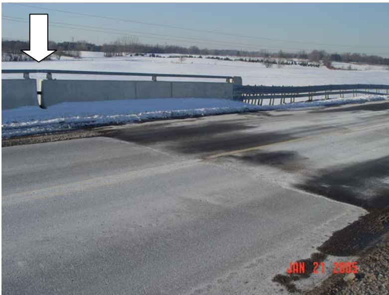
Figure 15.13: Concrete Barrier Cast Against RSS Preventing RSS Deflection.
