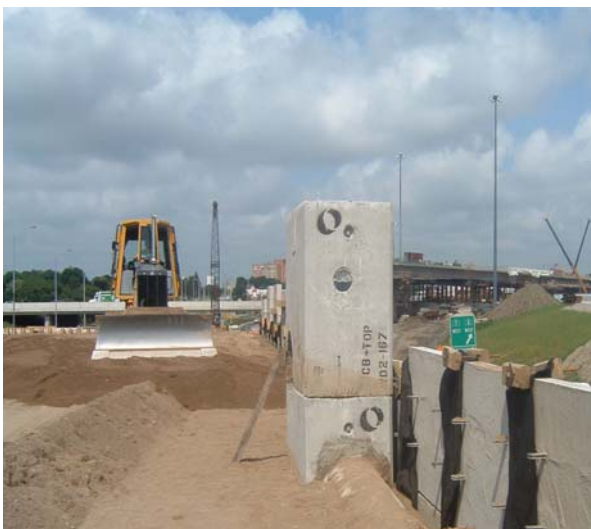
Figure 15.8: RSS Corner Element.
