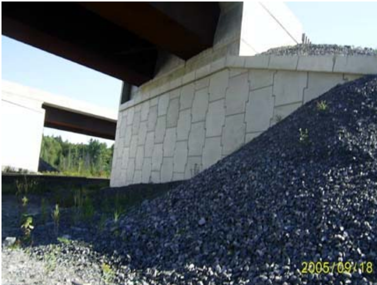
Figure 15.5: RSS False Abutment and RSS Wraparound Walls (Cast in Place Wingwalls Above).
