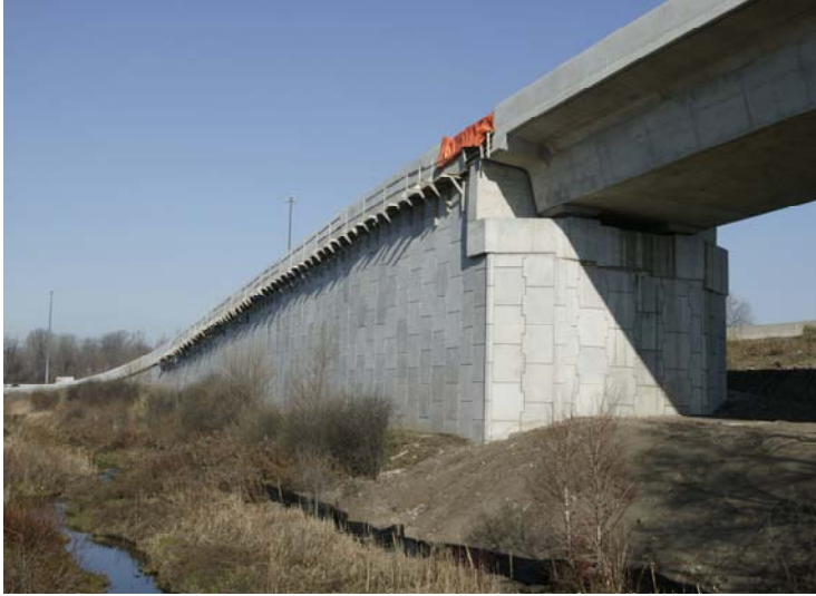
Figure 15.4: RSS False Abutment (Rigid Abutment with 2 Rows of Piles) with RSS Wingwalls.
