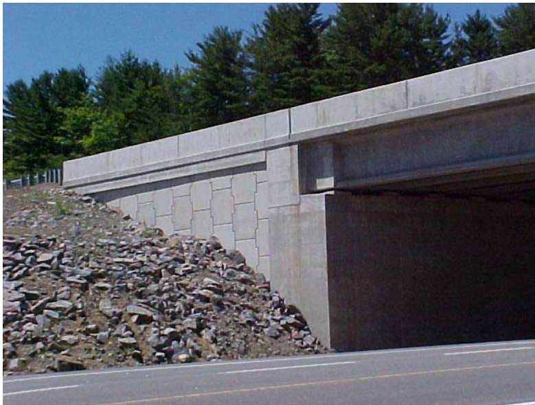
Figure 15.3: Conventional Abutment with RSS Wingwalls.
