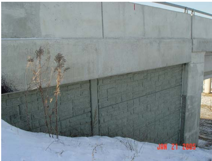
Figure 15.1: Concrete Integral Abutment with RSS Wingwalls.
