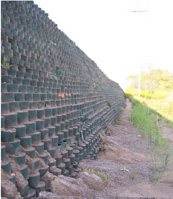
Figure 15.7: Armtex Ltd., Geoweb – Wall/Slope, Medium Performance, Medium Appearance Wall.
