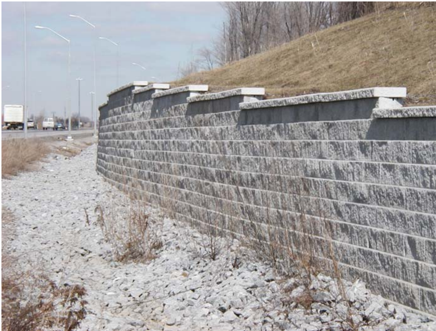
Figure 15.6: Tensar Earth Technologies Inc., Mesa – Wall/Slope, Medium Performance, High Appearance Wall.
