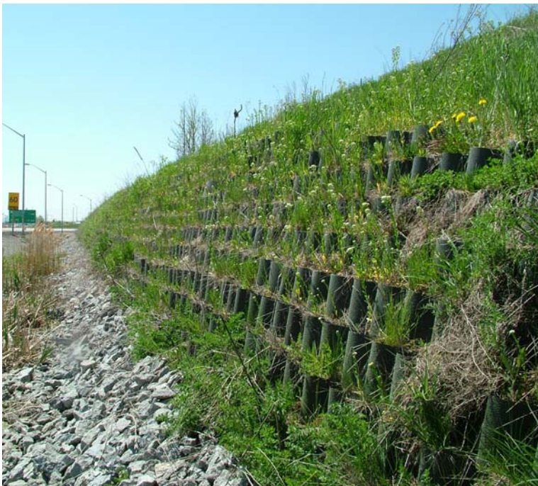
Figure 15.8: Tensar Earth Technologies Inc., Sierra TF (Terraweb) – Wall/Slope, Medium Performance, Medium Appearance Wall.
