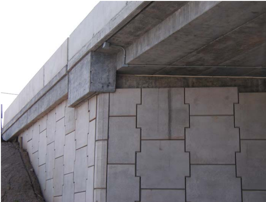
Figure 15.1: Reinforced Earth Company Ltd (RECO), Cruciform FA – False Abutment, High Performance Wall.
