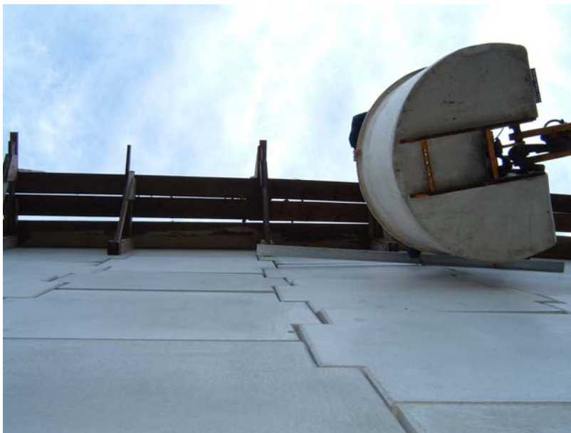
Figure 15.11: Cracking of Abutment due to Inadequate Allowance for RSS Settlement.
