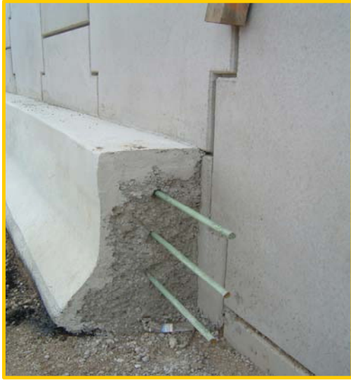
Figure 15.13: Concrete Barrier Cast Against RSS Preventing RSS Deflection.
