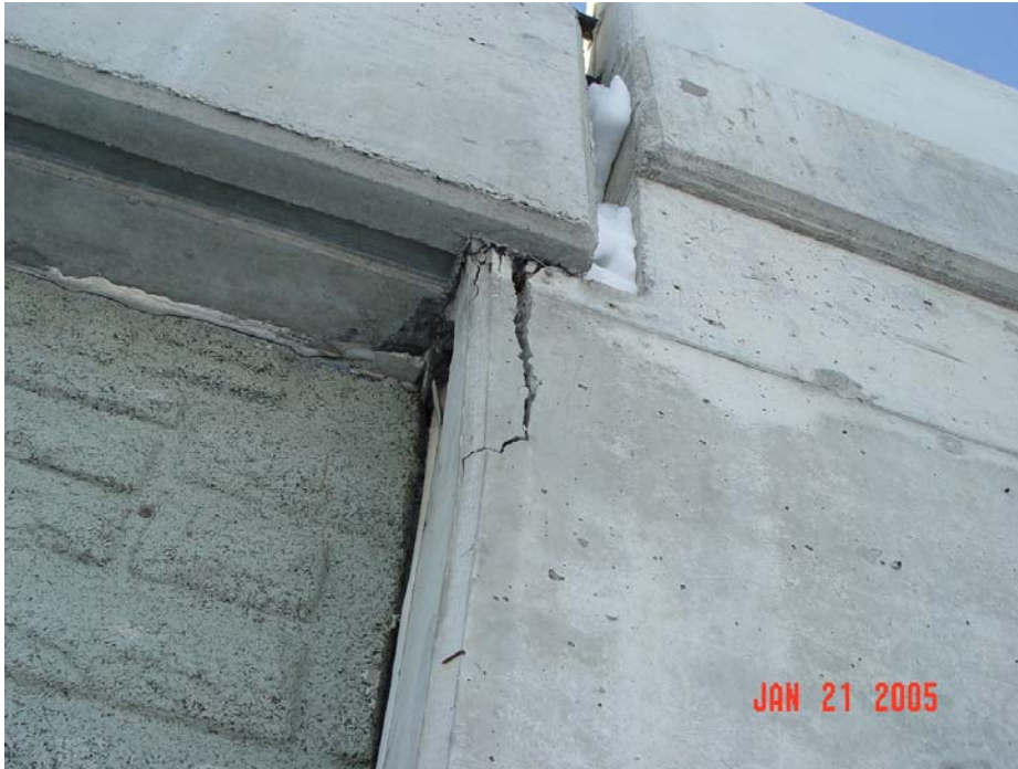
Figure 15.11: Cracking of Abutment due to Inadequate Allowance for RSS Settlement.
