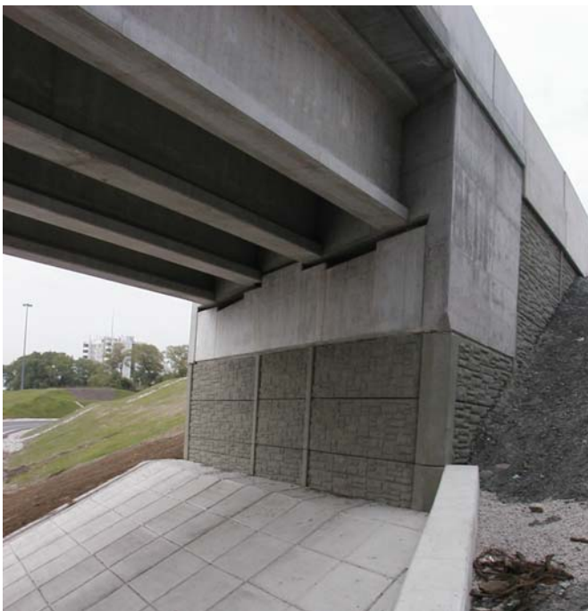
Figure 15.2: Durisol Inc., DFAS – False Abutment, High Performance Wall.
