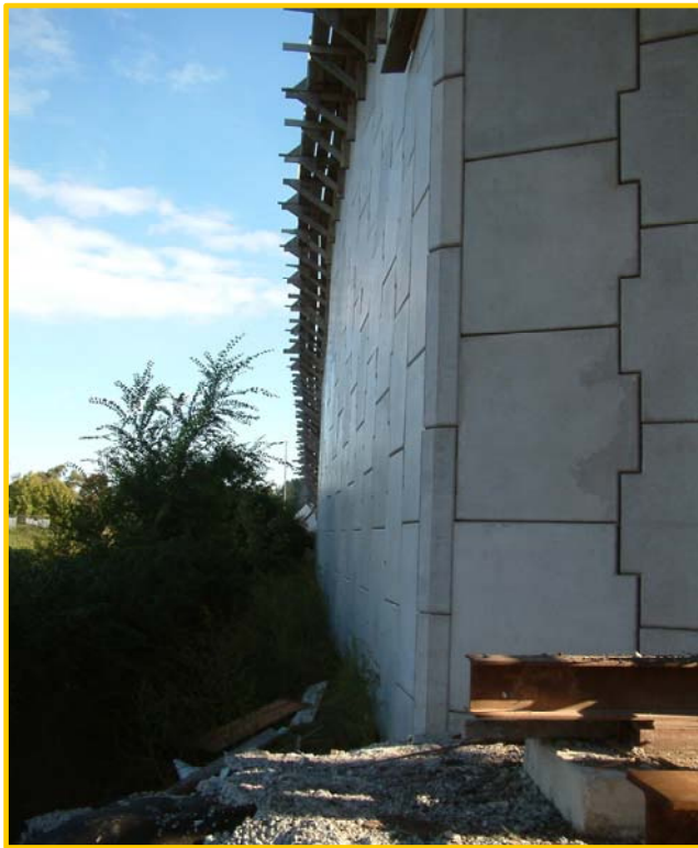
Figure 15.8: RSS Corner Element.
